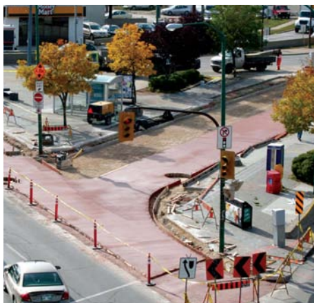
Construction au "Confusion Corner" – Winnipeg, Manitoba
